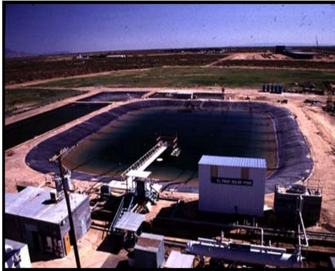
This photo displays a large scale salt gradient solar pond at the University of Texas at El Paso developed by John Walton and Andrew Swift.
