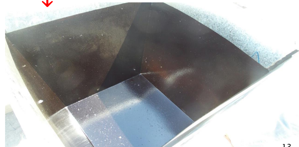
Coal tar Epoxy lining and double layers of Isolation glass wool (5 cm thick)
